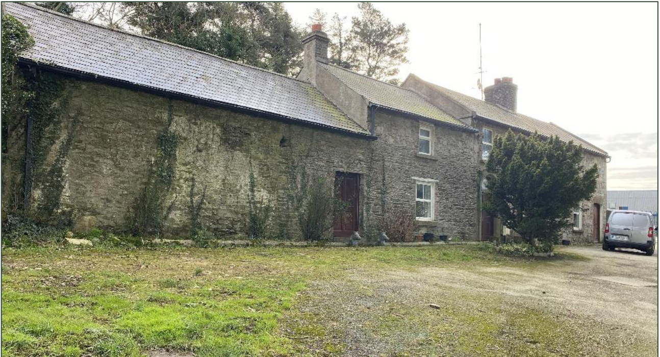
Figure 4.11: Buildings and artificial surfaces (BL3).
